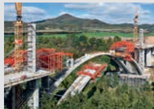
Bridge Formwork
